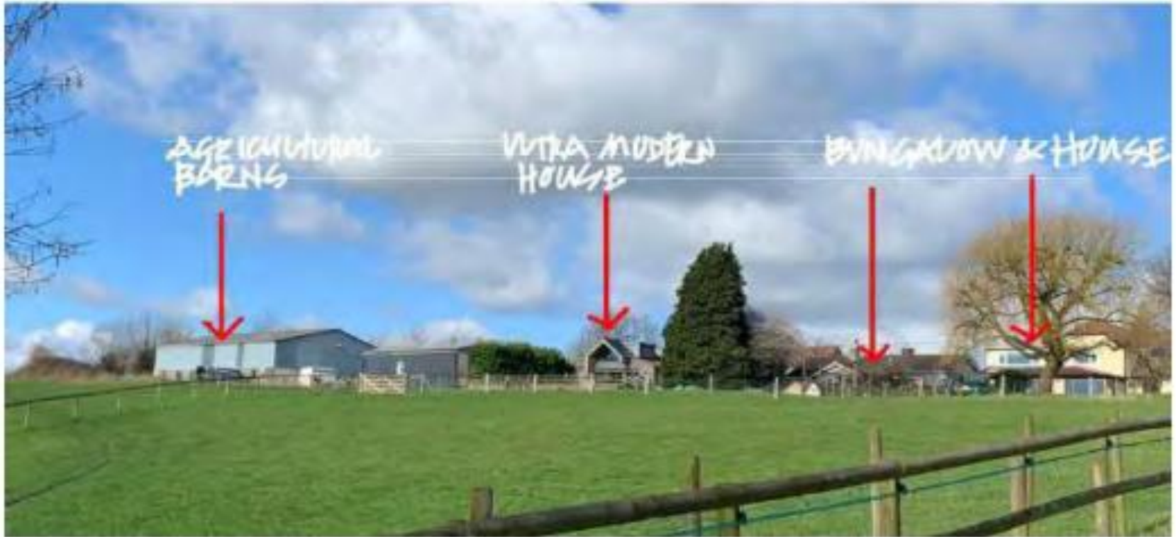
Above: Mix of buildings to the west of site off high street
